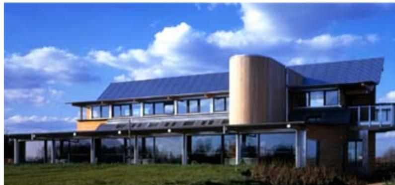
**Figure 3-53- Roof designed to adapt photovoltaic cells. Orientation of the building to make passive solar heating possible. ([www.penoyre-prasad.net](http://www.penoyre-prasad.net))**
