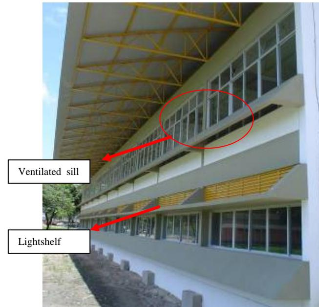
**Figure 3-20- View of the ventilated sill used in the building.**
