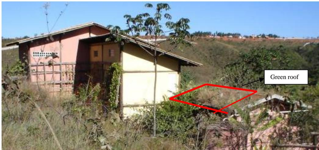
**Figure 3-24- Small or no windows on the Northwest facade and use of green roof.**
