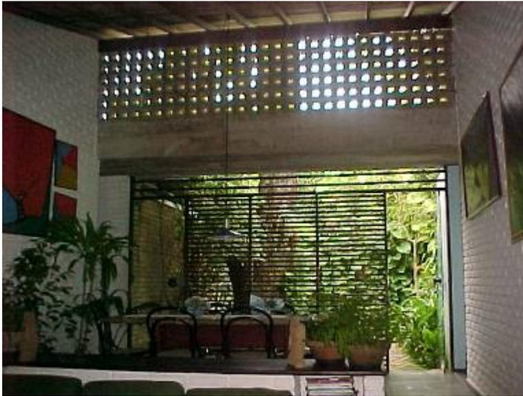
**Figure 4-13- House of Leonardo Bittencourt in Maceio, Northeast of Brazil. Openings to natural ventilation, extracting the over heat generated by the dark roof.**
