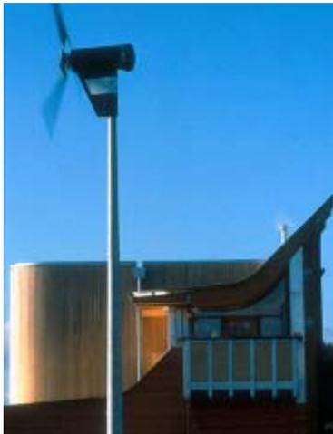
**Figure 3-52- Use of additional source of energy through wind turbine ([www.penoyre-prasad.net](http://www.penoyre-prasad.net))**
