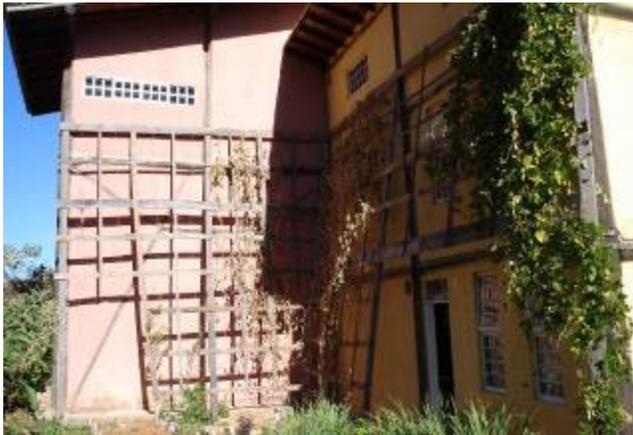
**Figure 3-25- Structure to protect the Northwest facade during summer.**
