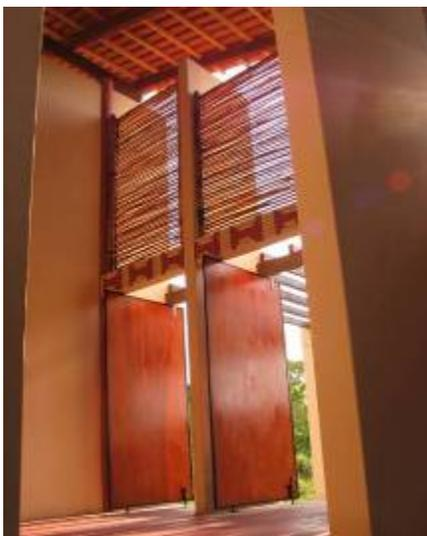
**Figure 3-27- Use of local materials. Permeability of the building. Use of “mobile” walls.**
