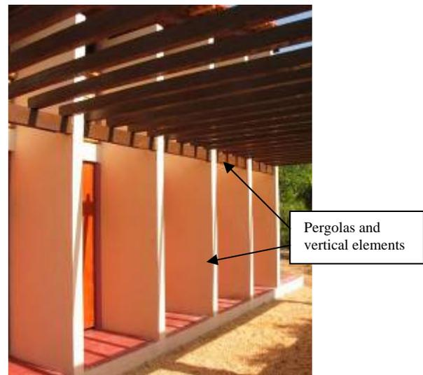
**Figure 3-28- Pergolas and vertical louvers to solar shading.**
