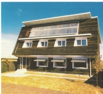
Figura 6: Saskatchewan Conservation House. Parker (2009)
