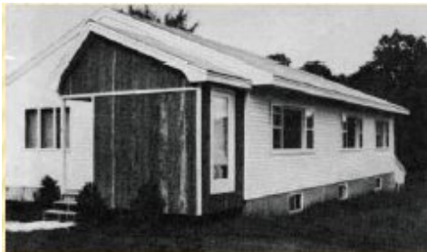
Figura 7: Foto da Leger Superinsulated House. Parker (2009)
