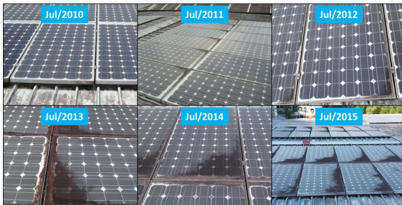
Figure 60: Progression of soiling accumulation in an unmaintained PV system due to a flat tilt angle (source: SERIS).
