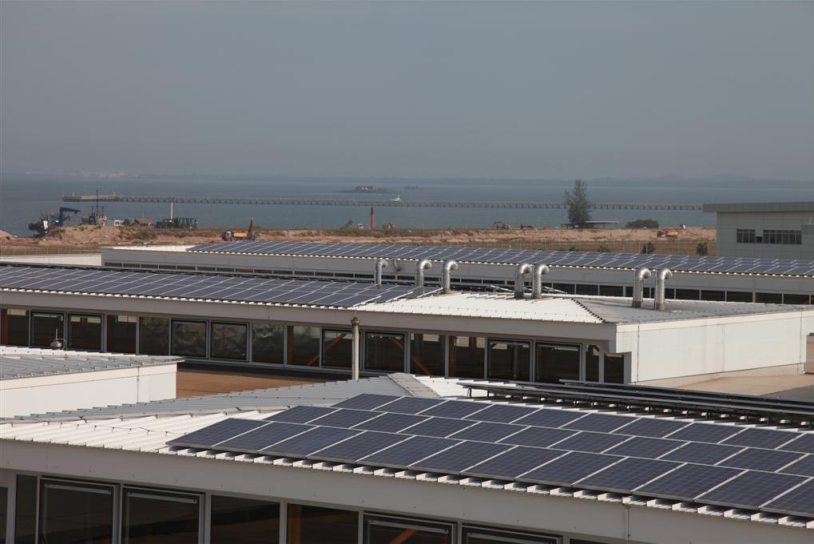
Figure 13: An industrial 300.4 kW p PV system at the REC facility in Tuas, Singapore with polycrystalline modules (NSR, 2013c).
