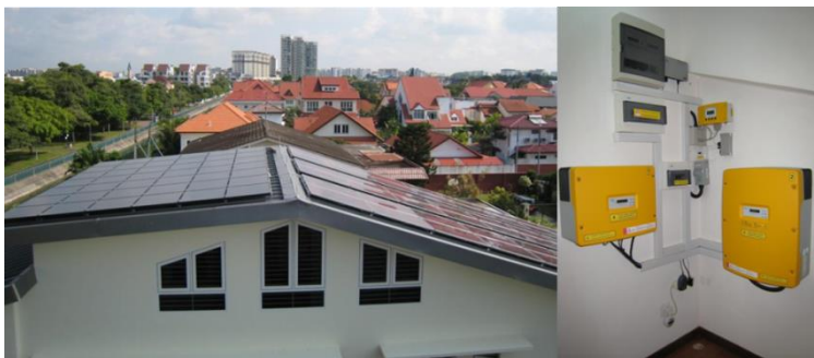
Figure 12: A residential 8.6 kW p PV system in Singapore with thin-film modules and two inverters (NSR, 2013c).
