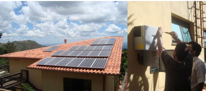
Figure 14: A 3.6 kW p monocrystalline PV system in a residence in Belo Horizonte, Brazil (SPB, 2012).
