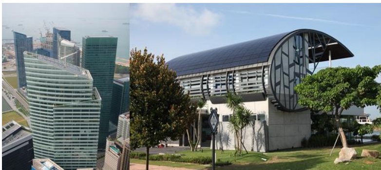
Figure 9: PV systems in Singapore exemplifying the urbanization of solar photovoltaics (NSR, 2015b).
