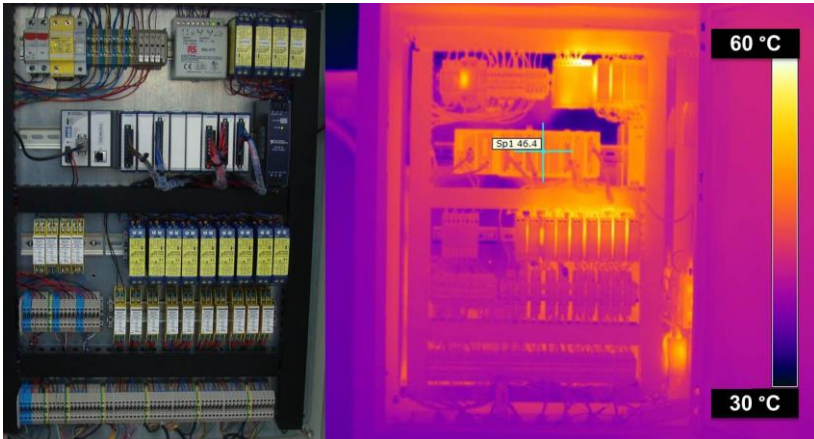
Figure 74: Thermography of a monitoring cabinet at around noon (source: SERIS).
