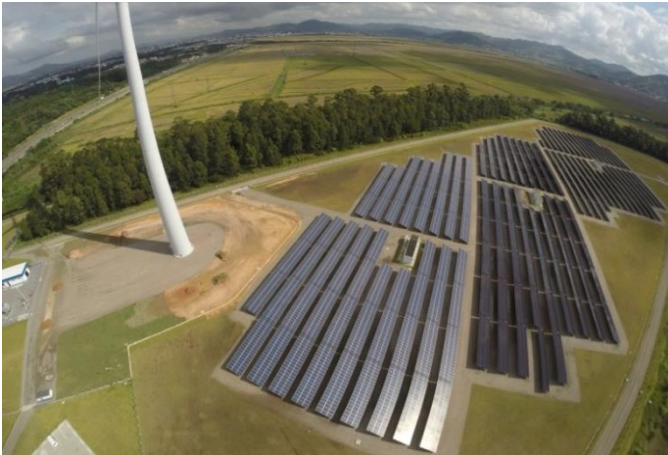
Figure 4: 3 MW p at the UFSC/Tractebel R&D facility in Tubarão, SC (Source: Fotovoltaica/UFSC).
