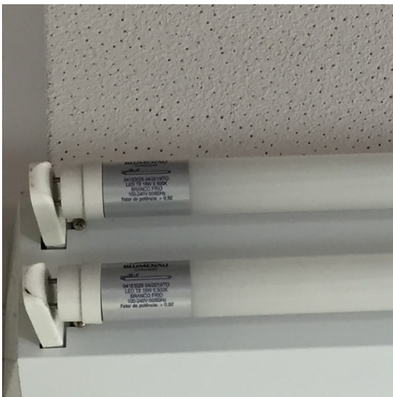
(c) Detail: Type of the predominant lighting system. A double LED T5 18W.
