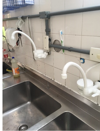
(f) Detail: water heater in the kitchen
