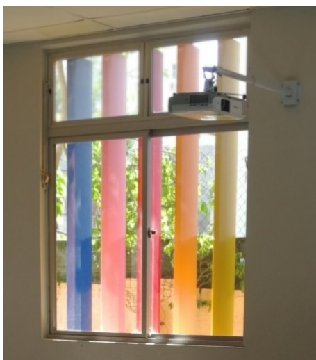
(e) Detail: Brises-soleil outside the some windows
