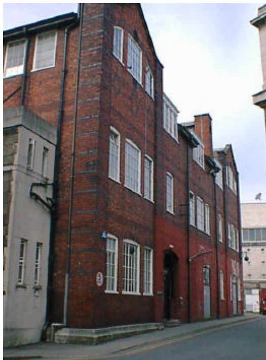
Figure 4.1. View of the Southeast façade of the Estates Services Building.
