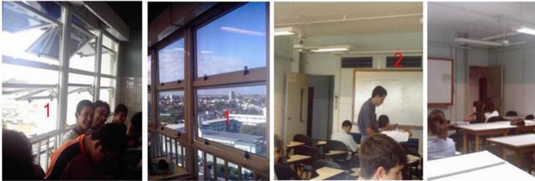
1: Sash windows 2: Venetians (iron).
