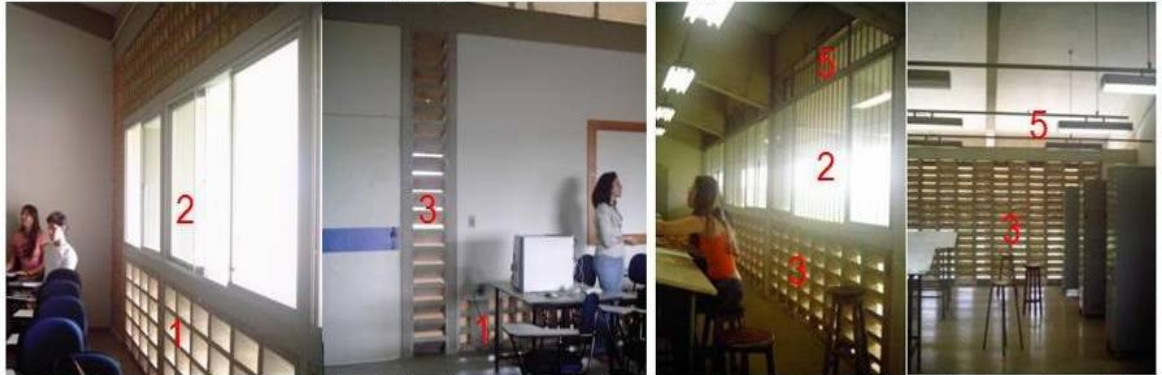
1: Perforated blocks 2: Sliding windows 3: Venetians (concrete) 4: Area for ventilation above the window 5: Open area for ventilation. a)
