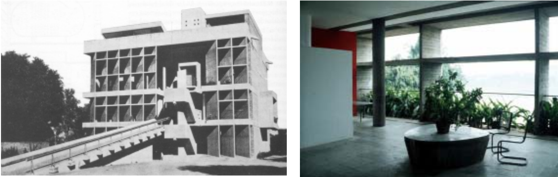
Figura 2-1- Mill Owners' Building. Ahmedabad (source: http://www.public.iastate.edu/~bfoth/mills.html )
